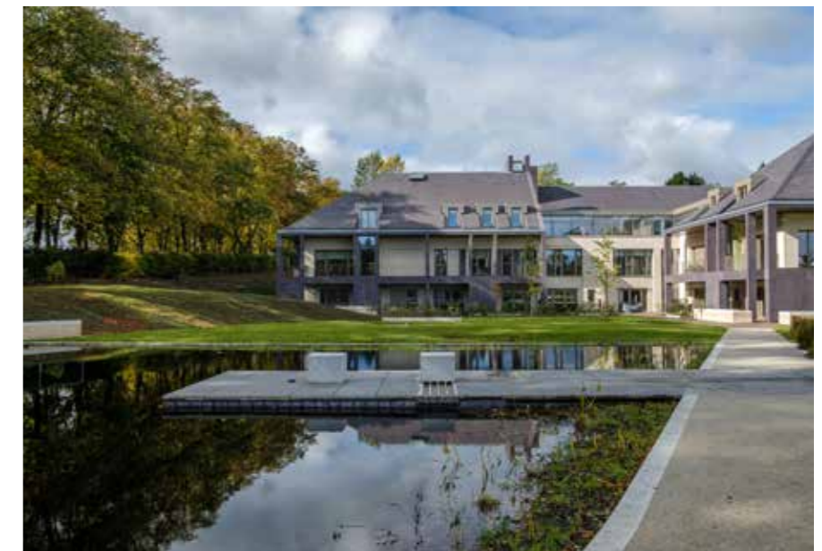
The pond at the new Prince and Princess of Wales Hospice delivers a calm focus for social activity and a wonderful setting for the new building, creating convivial space, creative and attractive functional water management and biodiversity. (erz 2019)
